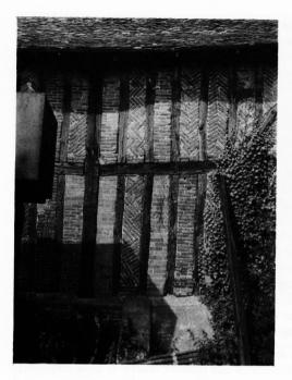
Fig. 10 Detail of the barn at New Hall. In the upper row of panels vents have been blocked with later bricks; in the lower row one panel has been filled with later bricks in reversed blocks pattern, and one with plain nogging. The others are mainly original.
