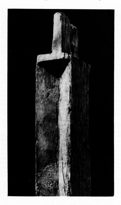
Fig. 16 A stud from the demolished manorial courthouse at Poole Farm. Great Yeldham, Essex, originally nogged in exposed face pattern. Note the smooth texture of original tooling in the V-shaped recess for mortar.
