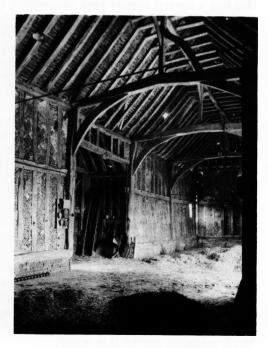
Fig. 11 Looking south-east in the barn at New Hall. The posts and studs are recessed to receive the mortar, and the recessed studs continue over the great doors. Brick Nogging
