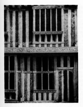
Fig. 15 Paycocke's, the right end of the main elevation. All the panels of opposed triangles are original; the parts disturbed by the construction of new windows and the doorway have been infilled with modern bricks in rectangular patterns.
