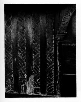
Fig. 12 Part of the north-east wing of Place House, Great Bardfield, Essex, built for William Bendlowes in 1564, with the carved corner post and original brick nogging in opposed triangles pattern.
