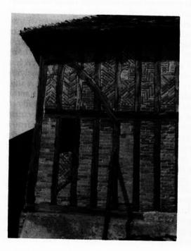
Fig. 9 Detail of the barn at New Hall. In the upper row of panels vents in alternate panels have been blocked with later bricks, but five patterns of original brick nogging are identifiable. In the lower row most of the original infill has been replaced by later bricks.
