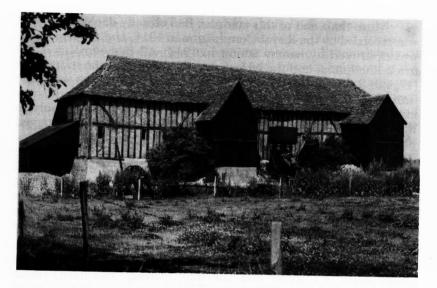
Fig. 8 The east elevation of the great barn at New Hall, High Roothing, Essex, built for Su Thomas Josselyn, 1554-62. The two midstreys are later additions. The brick nogging continues only half-way along the south end.
